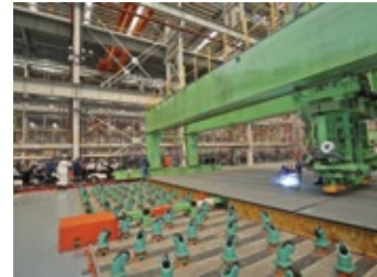
Opened a state-of-the-art steel structure fabrication workshop in Singapore, the largest of its kind in Southeast Asia
